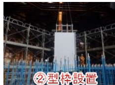
②型枠設置
